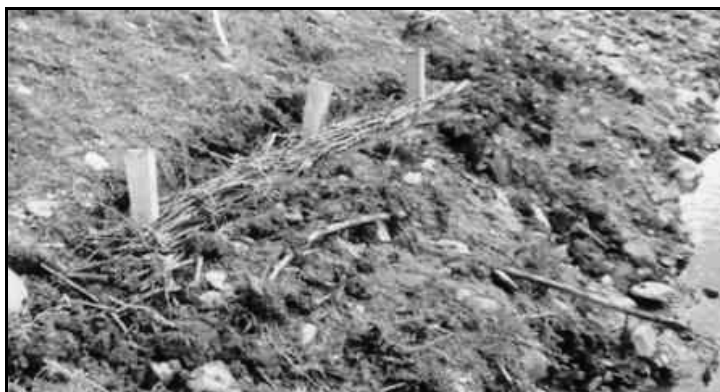
Live Red osier dogwood (shown above) and Streamco willow fascines were placed in shallow trenches parallel to the water's edge and staked in.
