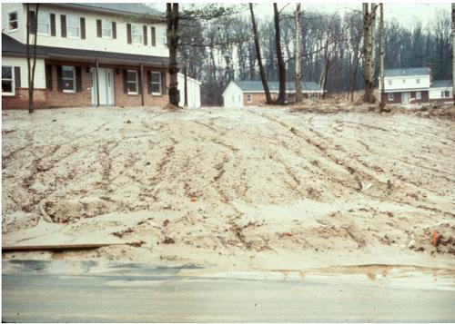
*Eroding soil from this construction site is transported in stormwater runoff and.....*
