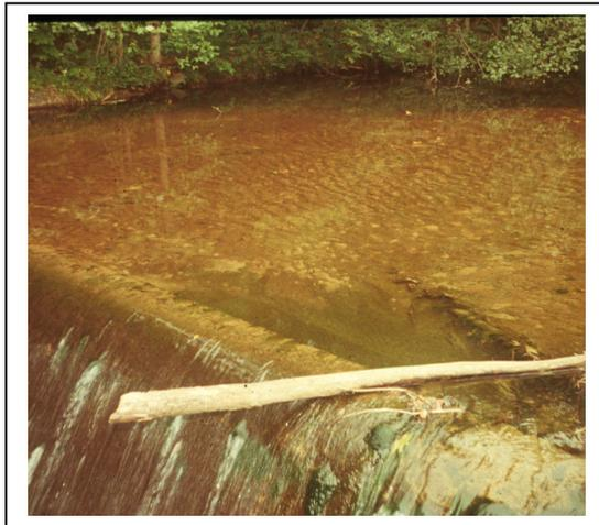
This water supply reservoir has fallen into disuse as a result of erosion and sedimentation due to road building for a subdivision that was never built upstream in the watershed.
